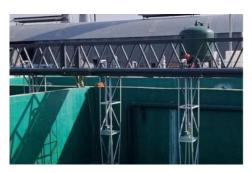
The main components of monorail underwater mud scraper are: transmission components, mud scraper trolley components, track components, guide wheel groups at both ends, tensioning device and electric control components.
